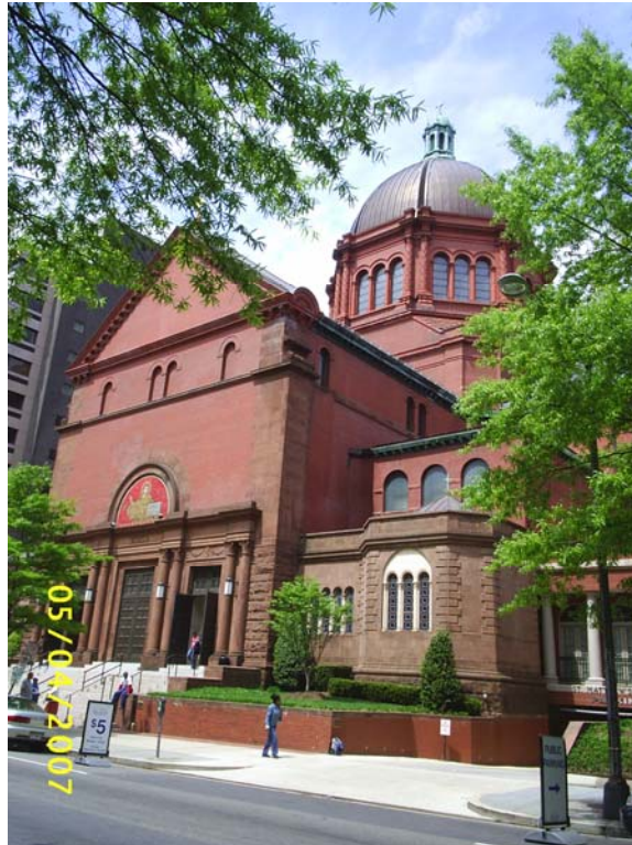
Front façade; St Matthew's Cathedral
