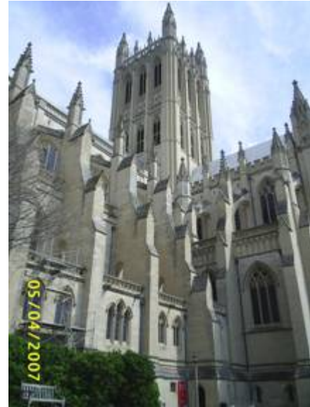
View of the flying buttresses.
