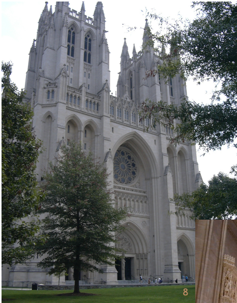
Side View - Main Entrance
