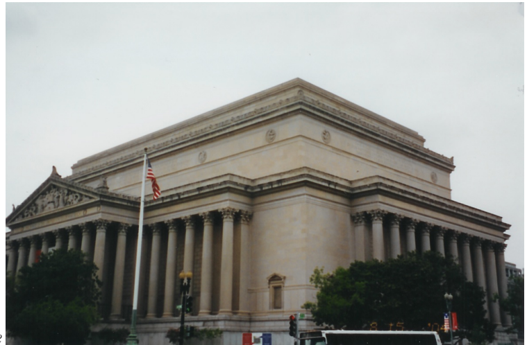
View from National Archives East Side
