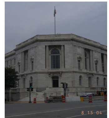
Russell House Office Building
